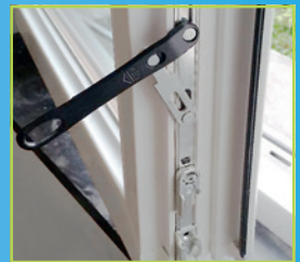
Reinforced secondary sash locking system
